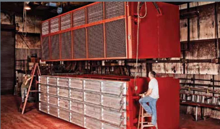
R Vertical coil, induced or forced draft, horizontal air intake and discharge, electric motor or engine driven fan.
